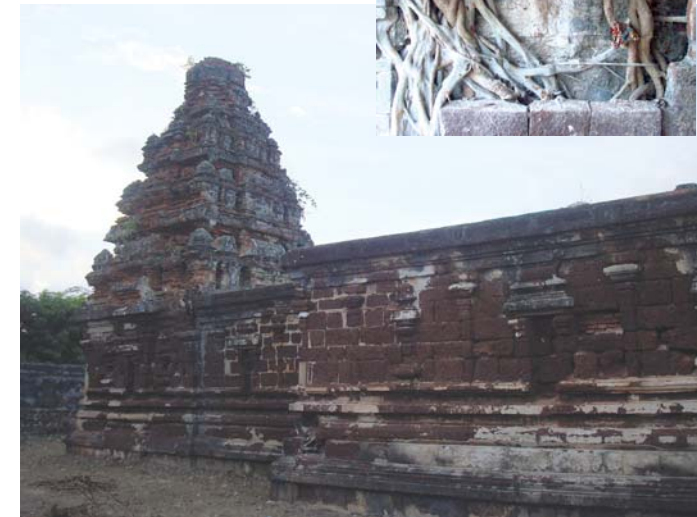
The Adinarayana Perumal temple of the Vijayanagara period and the roots of a tree tearing its walls open.
