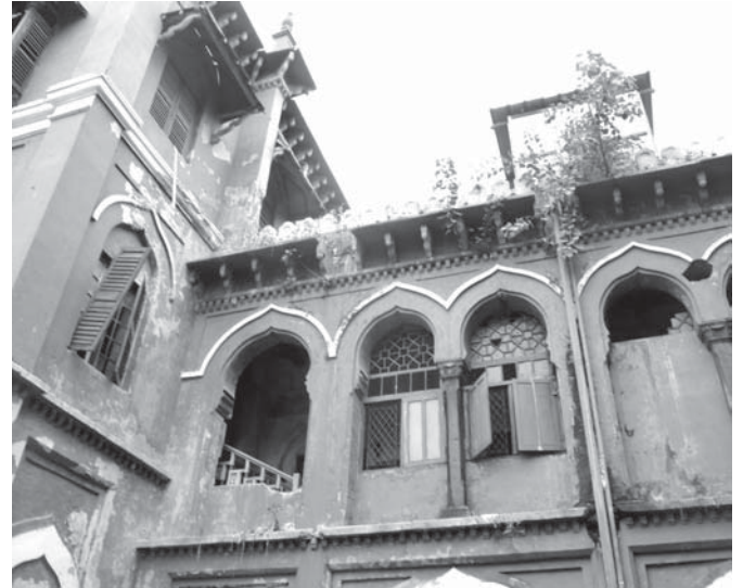
Khalsa Mahal awaiting restoration!
