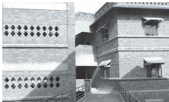
Abacus School, Chennai, the work of Laurie Baker, building in the traditional way.
