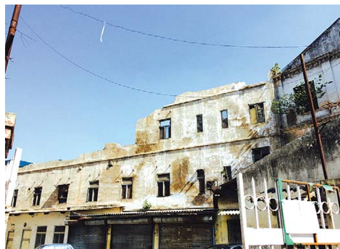
D'Angelis/Bosotto Building, now under the wreckers' hammers.
