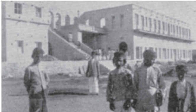
The Besant College buildings coming up.
