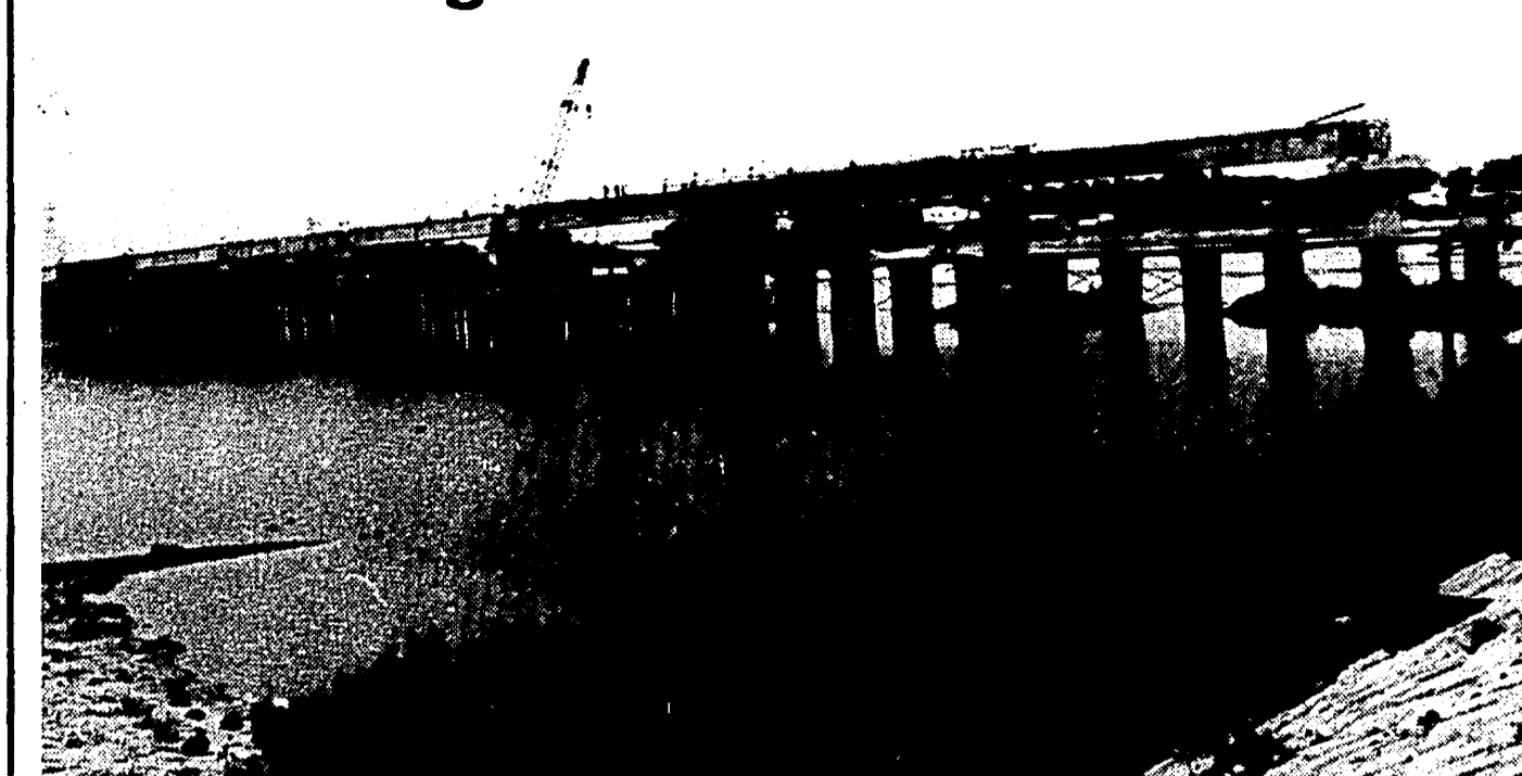
The National Highway Authority of India is in the process of constructing a bridge over the Porur tank to connect the 19 km phase one Tambaram-Poonamallee bypass. The U.P. State Corporation Limited is building the bridge. Work on the 462-metre bridge begun in May 1999 is expected to be completed by July 2000. The bridge which will rest on 16 pillars, sunk upto a depth of about 7-8 metres is founded on well foundation. A steel bridge has also been temporarily put up to facilitate easy moving of the machinery and workforce. The bridge when completed will have a 12-m carriageway inclusive of pedestrian space. This is the U.P. State Corporation's second bridge in Tamil Nadu after the first bridge at Chengalpattu.
