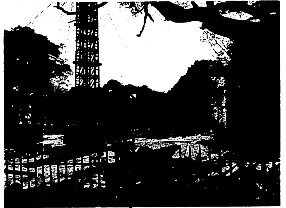
Pile-driving equipment brought in to start work at the Connemara Library-Museum Complex on Pantheon Road. This equipment will threaten both buildings, it is feared. (Photograph by RAJIND N CHRISTY.)
