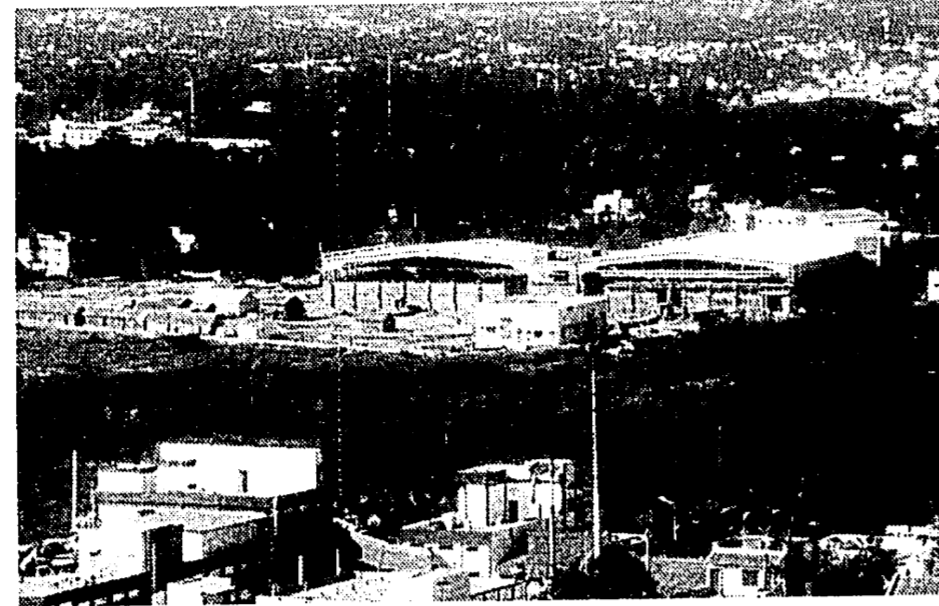
Work in progress at the Exhibition and Convention Centre being built in Nandambakkam. Two buildings are expected to be inaugurated in time for the Leather Fair at the end of January 2001. (Photograph by RAJIND N. CHRISTY.)
