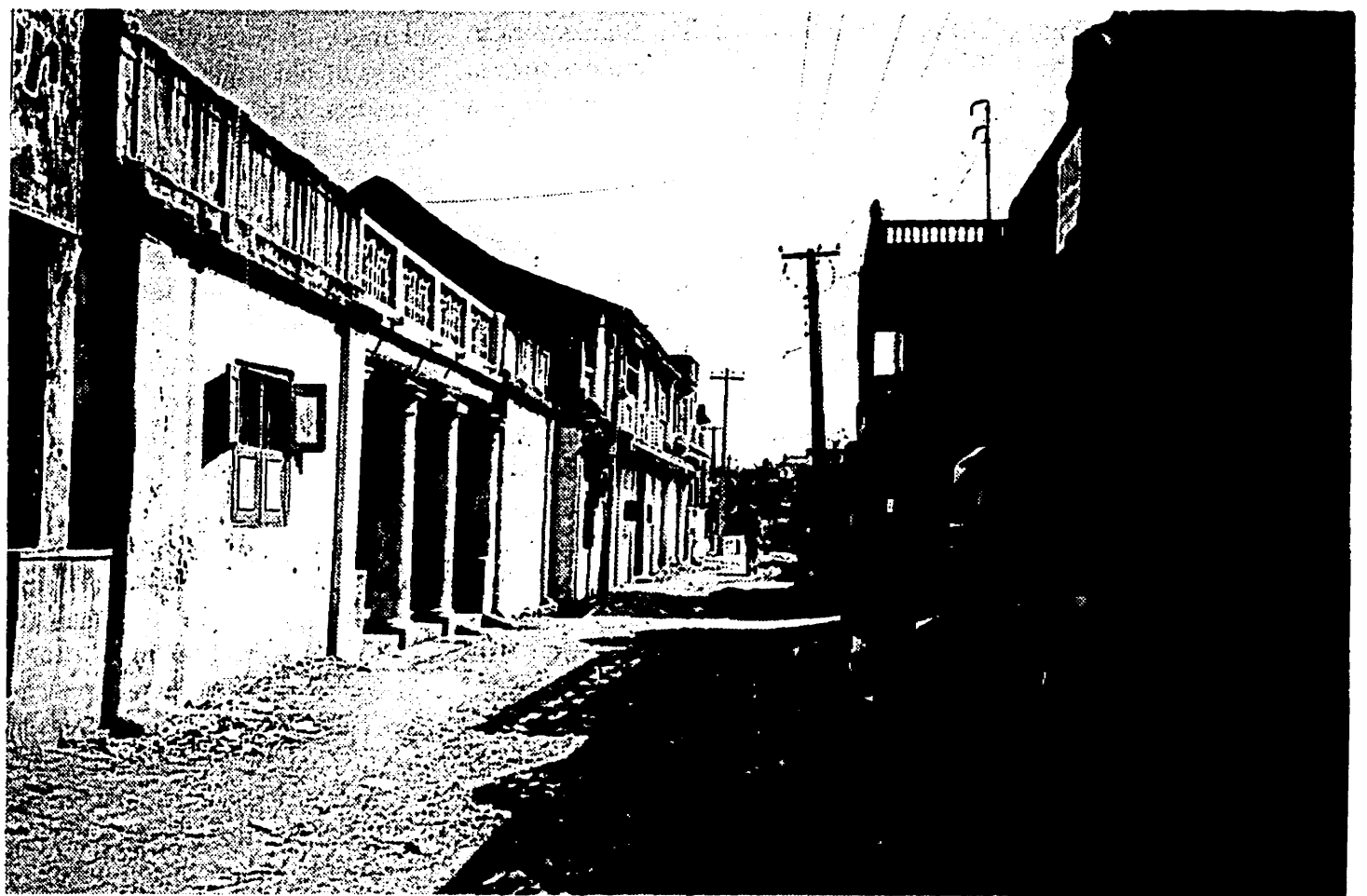
A Pulicat street, with some of the town's century-old houses. (Photograph by RAJIND N CHRISTY.)
