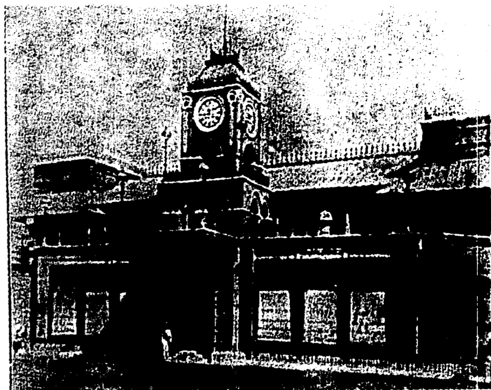
Our OLD is the home of P. Orr and Sons as designed by Robert Chisholm and built in 1873. Its clock tower was once connected to Madras Observatory and signalled standard time to the residents of the city.
