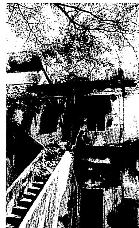
The rear of Capper House, with tree growth unrestrained.
