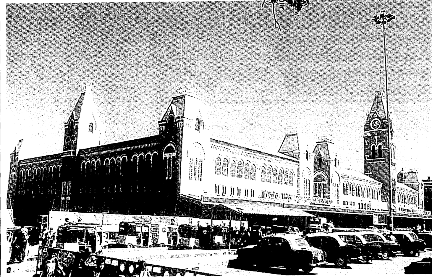
Our OLD this time (above) is the Central Station, designed by Robert Chisholm and built by George Hardinge between 1873 and 1878, and its extension built by Southern Railways, both reflecting Chisholm's 'County Cabs' tops, characteristic of combined western country and Kerala architecture that Chisholm used in many of his buildings in the Madras Presidency.
