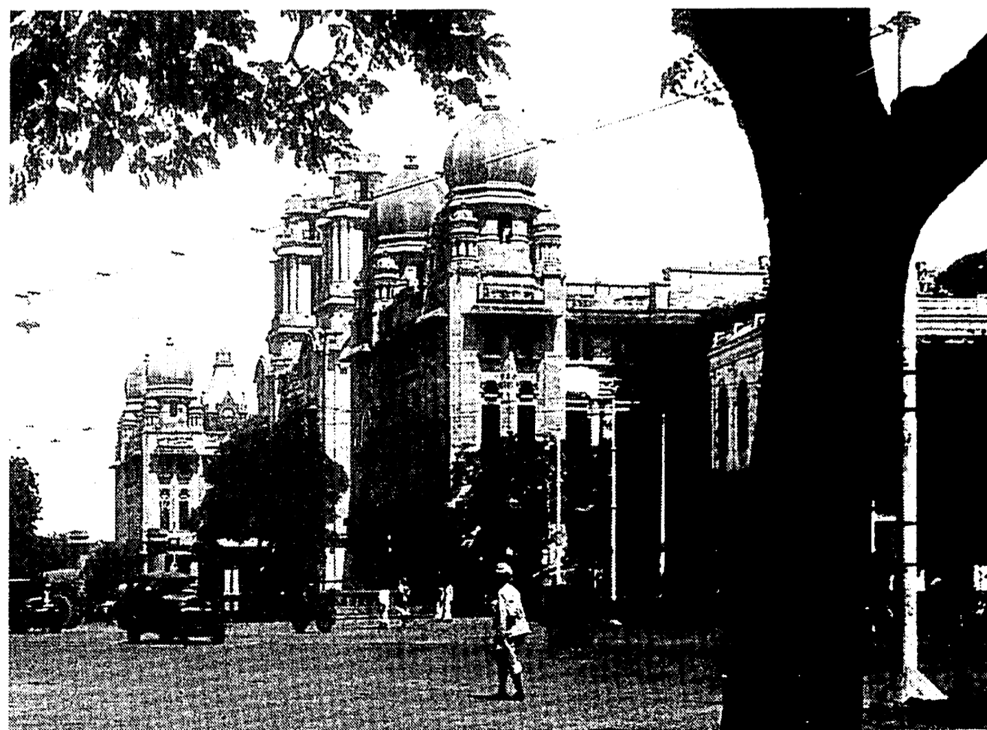
The present Southern Railway Headquarters soon after it was built as the headquarters of the Madras and Southern Mahratta railways.
