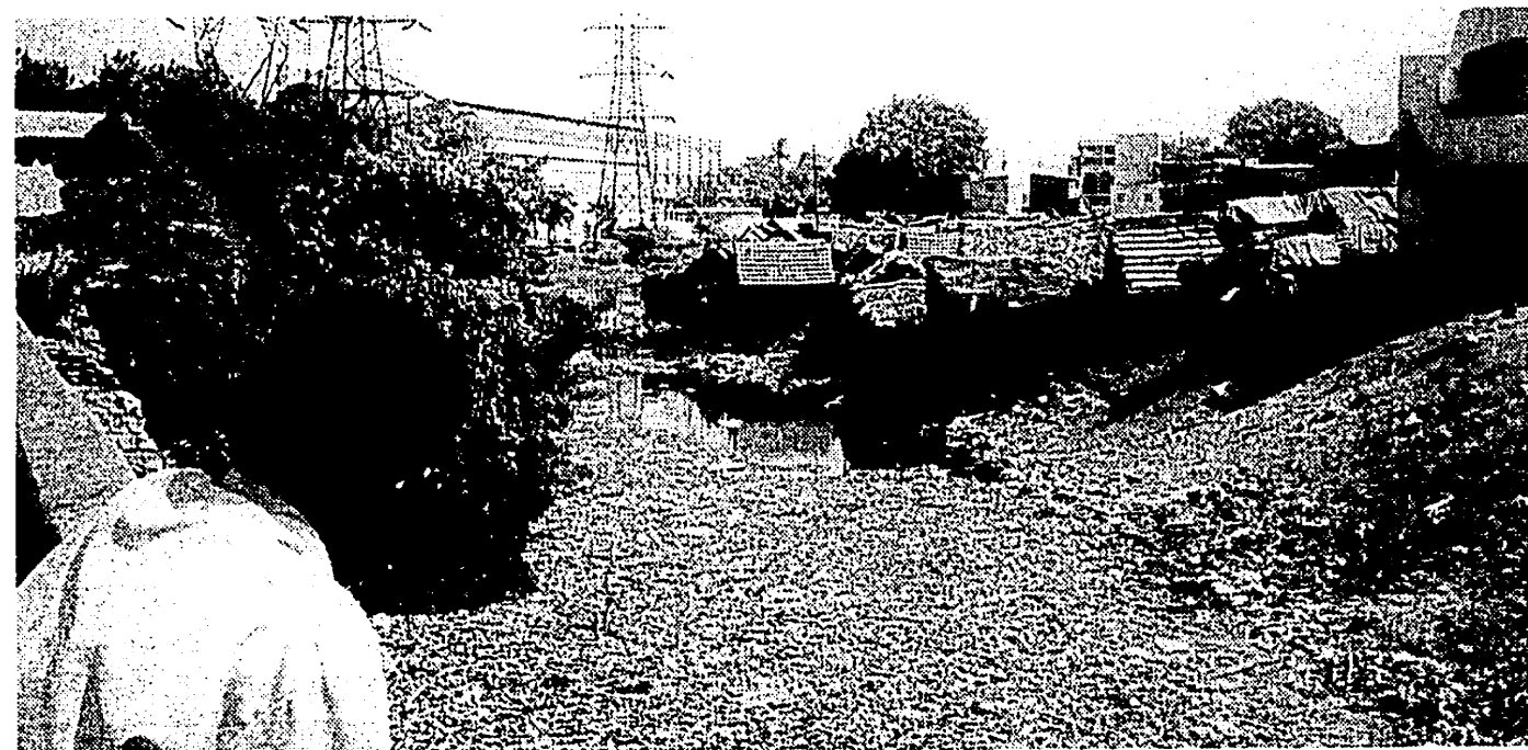
... and clogged waterways ensure the mosquito menace remains with us.
