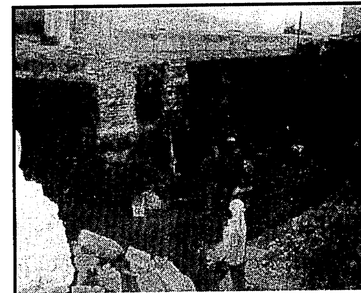
Excavation under the Basilica that could endanger the structural safety of a historic heritage building.
