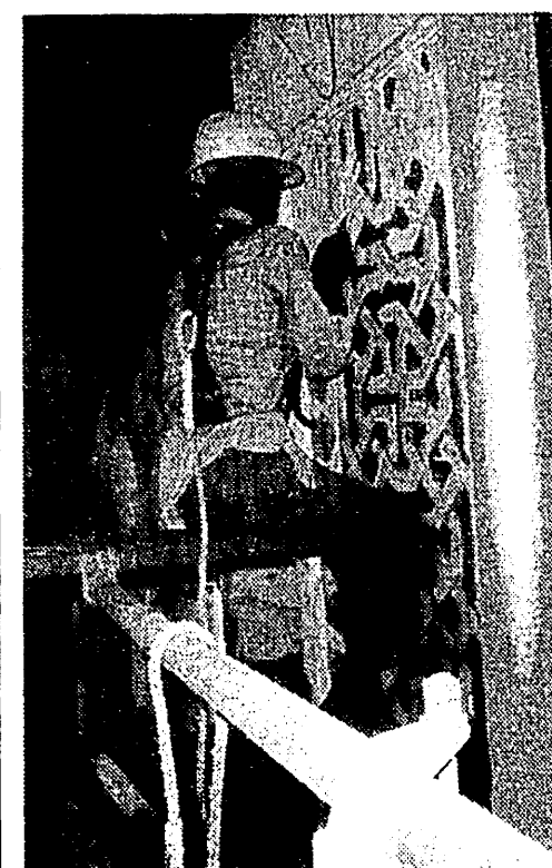
The frescoes being restored at Senate House as part of the restoration supported by the Chennai Willingdon Corporate Foundation.
