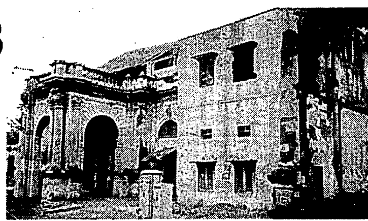
The Royapuram Railway Station.
