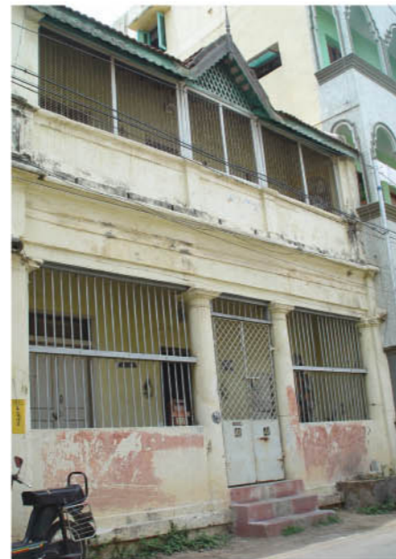
41 Nadu Street, the home of V. Sundaram Iyer. (Picture courtesy: MYLAPORE TIMES.)
