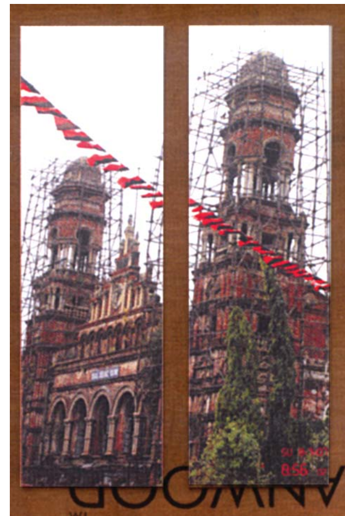
Kardy under renovation. Photograph by Prasanna Kumar N.
