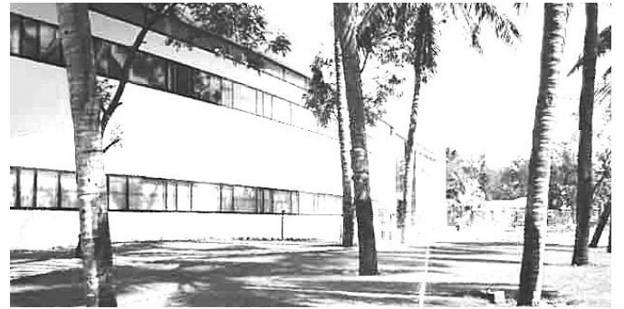
The 'golden' Grundfos green building.
