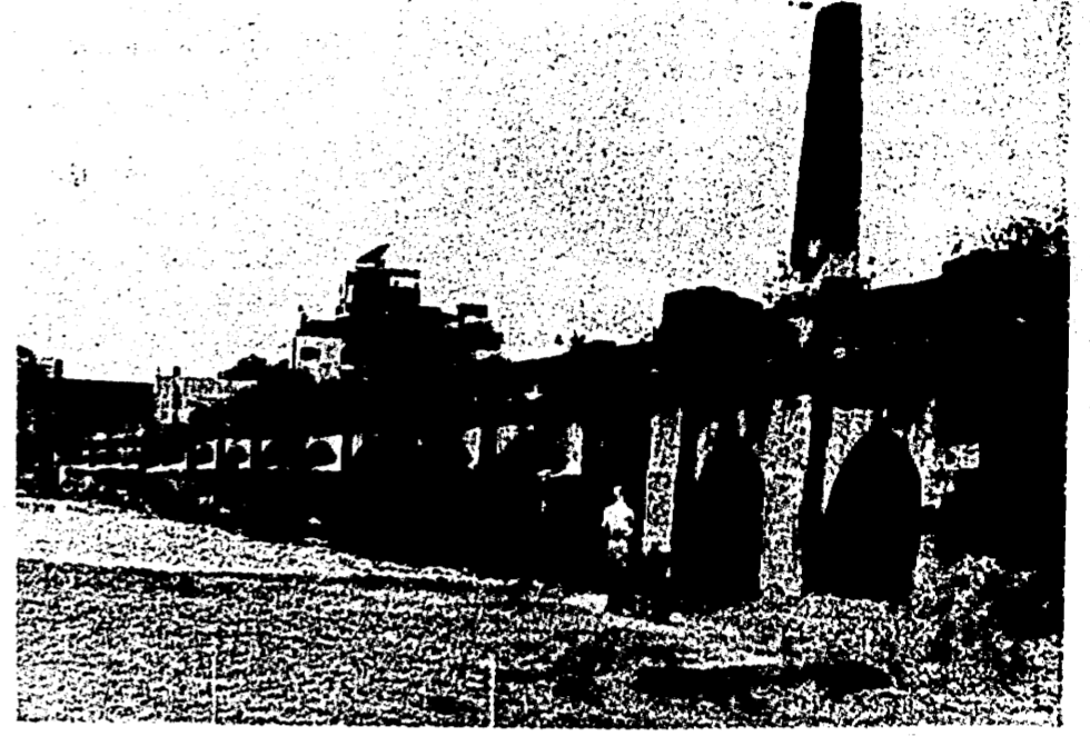
The Elphinstone iron bridge in Adyar is now shorn of its girders, sold several years ago to the highest bidder and not to a Raman-come-to-town. Now overgrown with shrub, the forlorn bridge awaits someone finding new use for it. (Photograph by K N CHARI)
