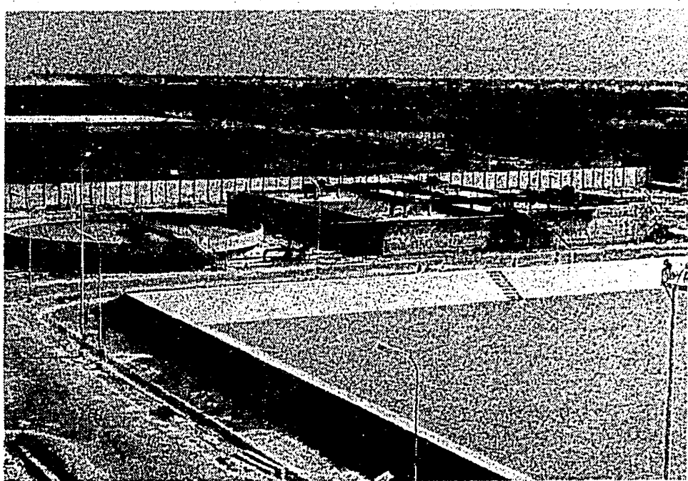
MRL's water treatment plant where sewage water is converted into water suitable for industrial use.
