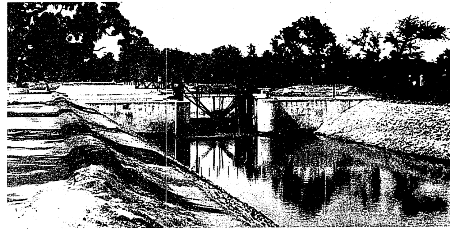
...OLD is a scene along the Buckingham Canal in the Forties. The Canal used to be navigable in those days and was an important transport system as the accompanying two-part feature narrates. And controlling the flow of water were locks like this one. Of such locks none are left... and the Canal is, if anything, worse than even today's Cooum!
