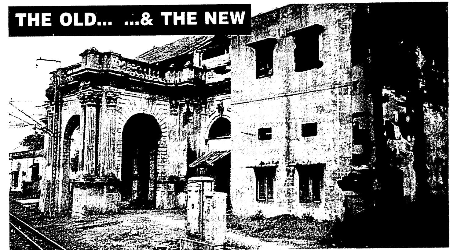
The NEW: The Royapuram Railway Station today... a dilapidated structure whose entrance alone shows vestiges of its ancient grandeur in its fluted Corinthian pillars.
