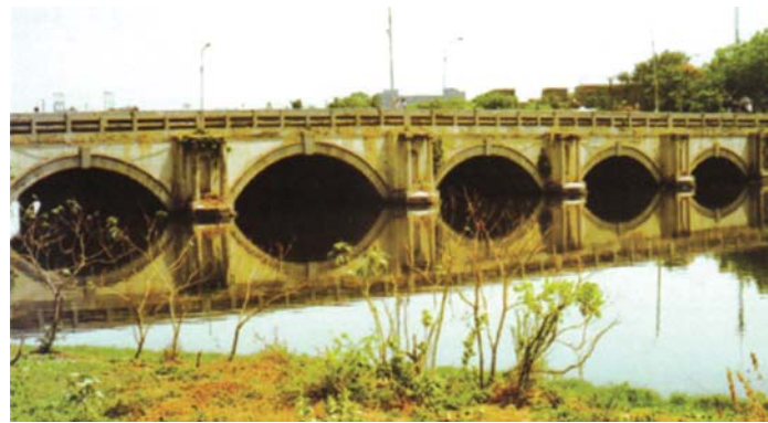
St. George Bridge, Mount Road, River Cooum.
