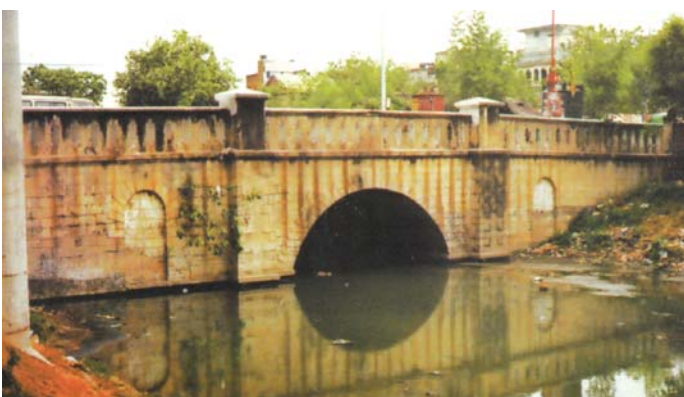
M.K. Amman Koil Bridge, M.K. Road, Buckingham Canal.
