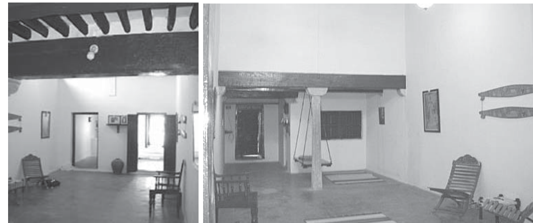
The restored, refurbished hall.
