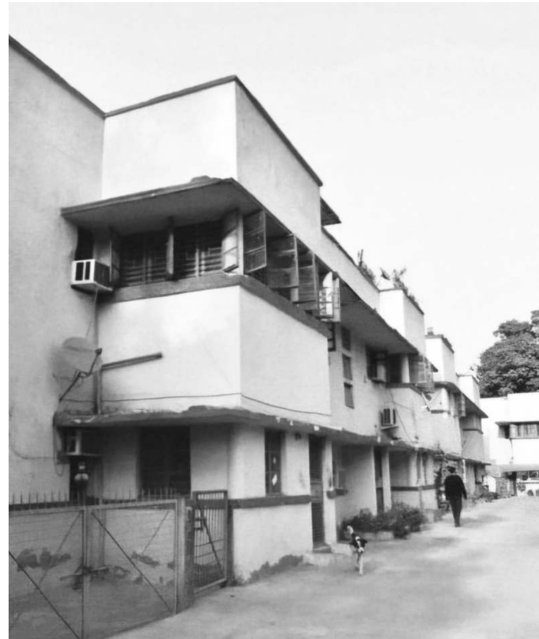
Government built houses like these in which numerous Tamil families lived for long years, thanks to the government jobs held by the head of the family. Many of these houses have been now razed by the current government to make way for high rise apartments.
