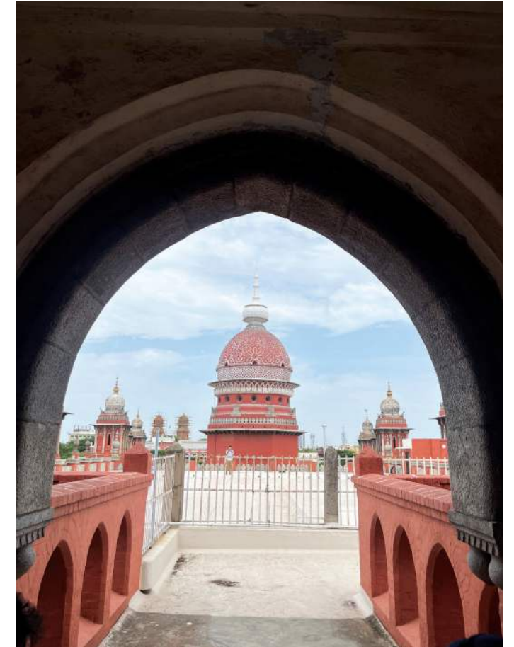
Beautifully framed West Block dome with a uniquely shaped finial.
