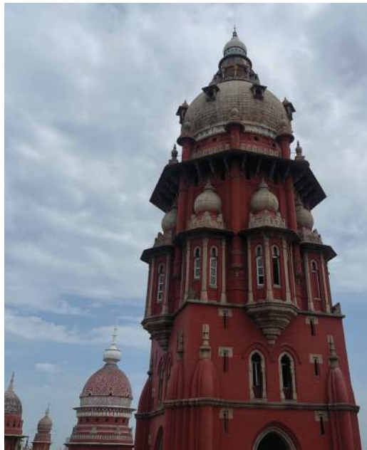
The piece de resistance of Madras High Court is the main 'lighthouse' dome.
