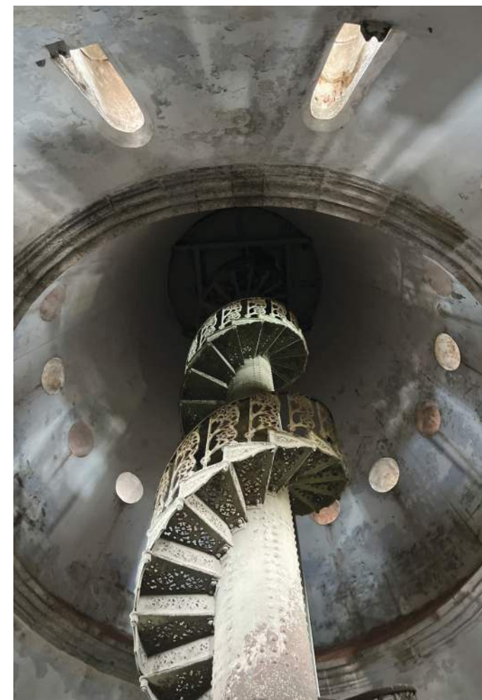
The spiral staircase leading to the lighthouse of Madras High Court.
