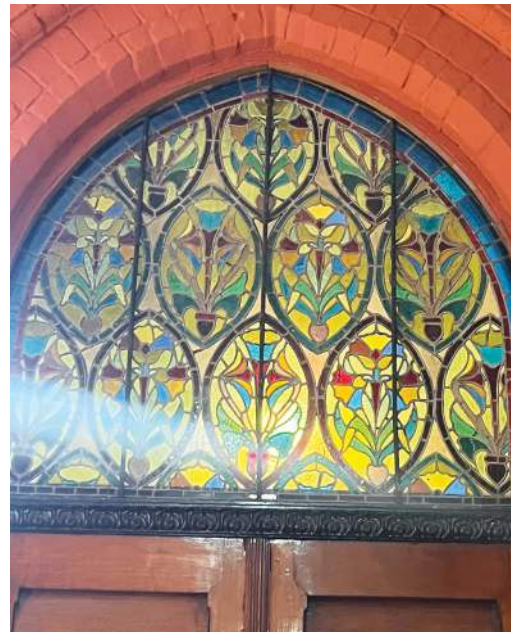
Spectacular stained glass doorways to courtrooms.
